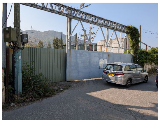
2 – General view of the Western Parcel of the Subject Site
