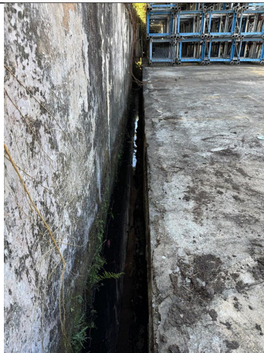
4 – Existing 300UC along the southern site boundary of the Western Parcel of the Subject Site (2 of 2)
